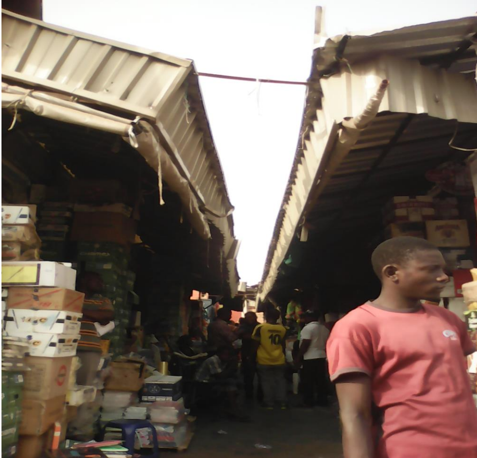
Plate IV: Lock-up Shop Buildings in the Market in FCT with Inadequate Spaces between them (Source: Researchers' Field Work, 2020).
