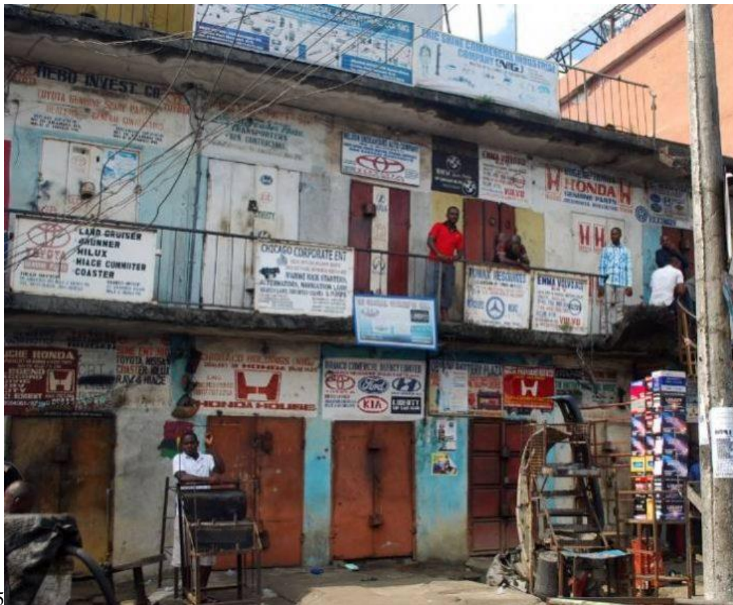
Figure 4. Ikoku Spare Parts Market showing the Use of Steel Panel Doors in its Construction. Source: Twitter, 2018 ( https://twitter.com/AskPHPeople/status/1050743414185189383 ), Retrieved on 08-12-2022.
