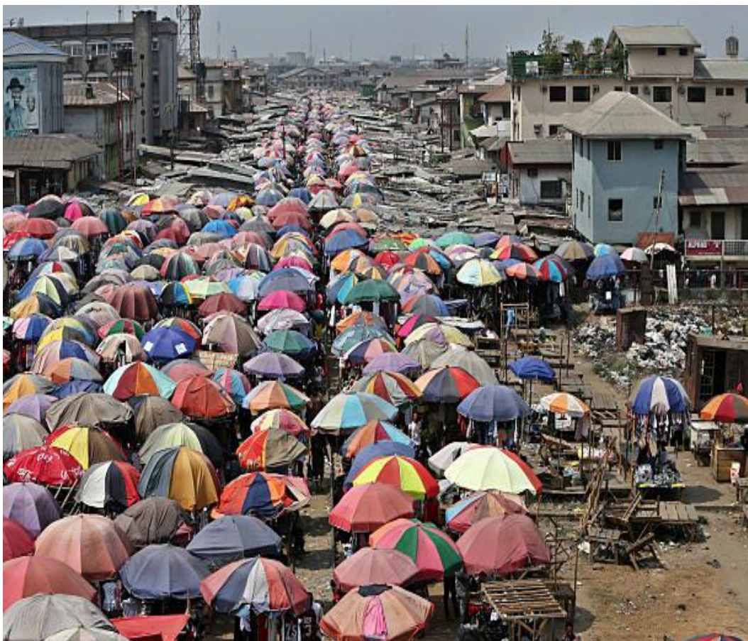
Figure 3. Mile 1 Market showing the Use of Steel Panel Doors; Window Panes and their Aluminium Frames in its Construction.
